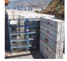
17 Andenes Reefer 17 Reefer connection structure
