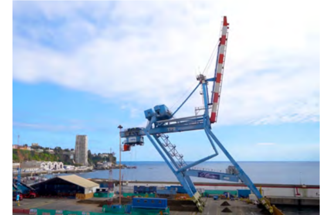
Controlled Collapse of a Gantry Crane.
